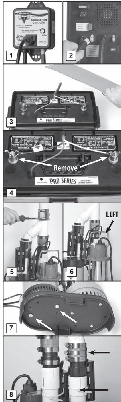
5. Slowly loosen the no hub coupling on the top of the combination pump assembly to separate the pipes. The water trapped in the pipe will pour out into the sump as the no hub coupling is loosened.
