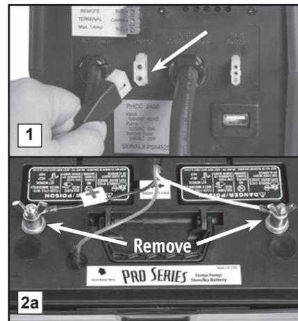
1. Check the pump plug in the back of the unit to make sure it is firmly connected. Check the pump wires to make sure they are connected securely to the pump plug. Check the rest of the pump wires for any possible breaks.
