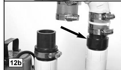
13. Reconnect the pipes to the Y-assembly and line up the pipe on the primary pump parallel to the pipe on the backup pump. Tighten the no-hub connectors.
